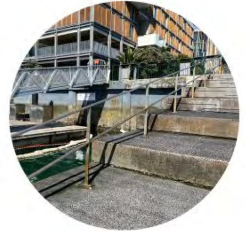
004. Existing handrail is easily climbable and allows jumping off the edge of the steps.
