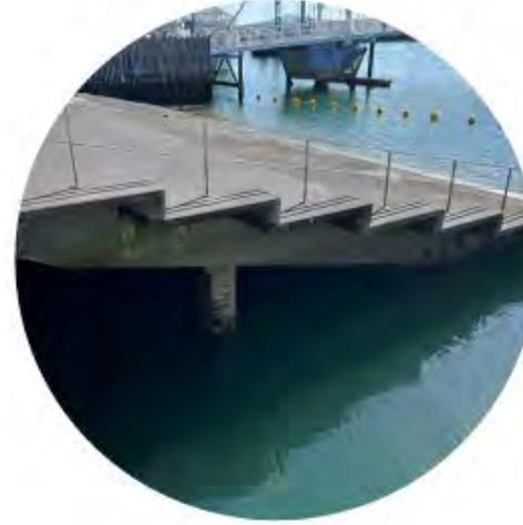
003. Open underside of Tidal Steps presents a potential hazard if swimmers enter beneath (current, low lighting etc)
