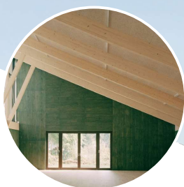
Glulam Roof structure and clerestory daylighting:
