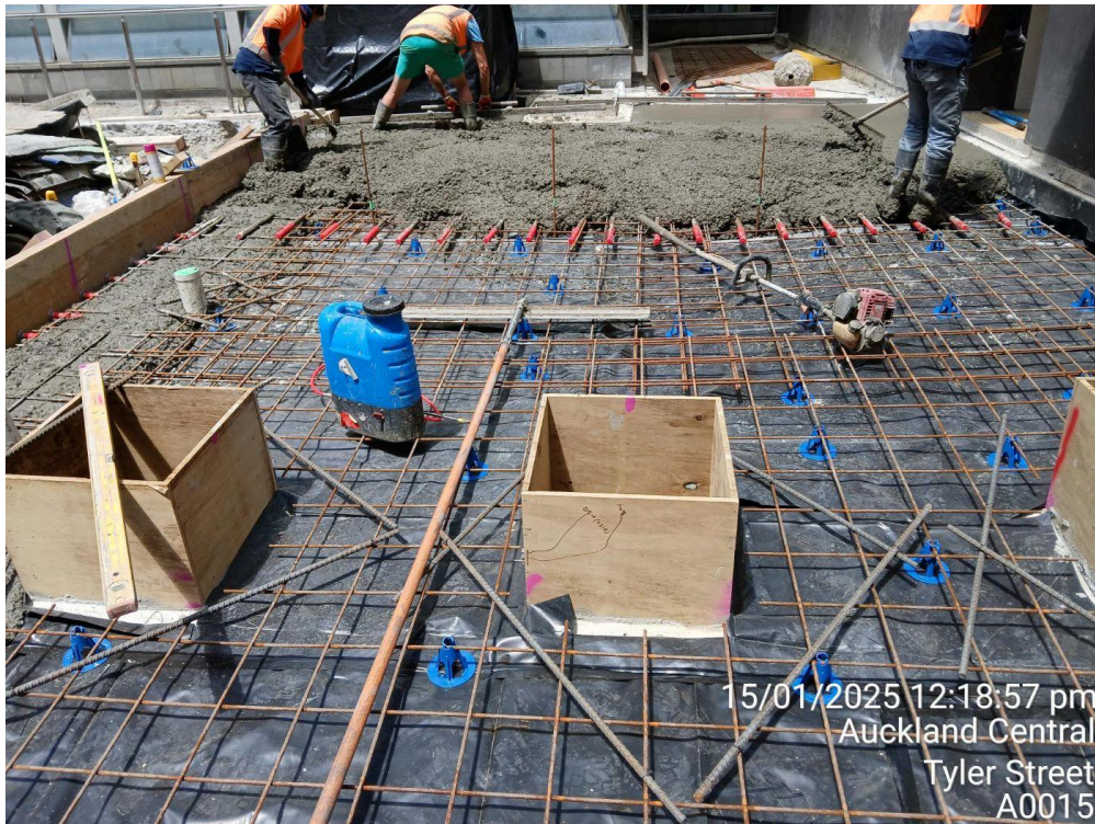
Image: preparation for concrete pour within Waitematā plaza, January 2025
