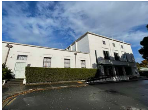
NORTHERN FACADE - WAR MEMORIAL HALL
