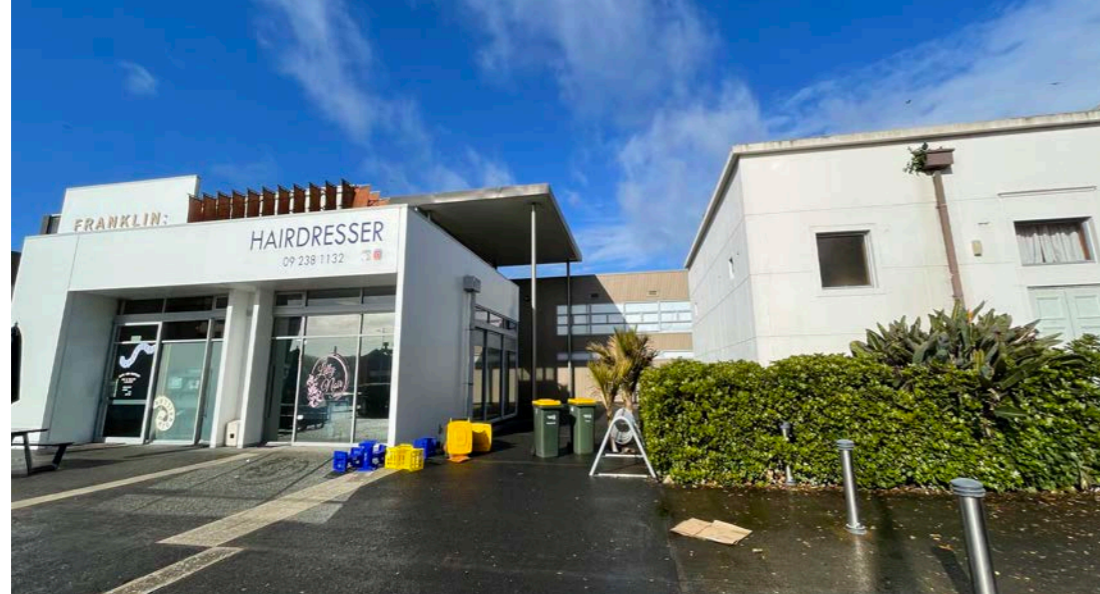
NORTHERN FACADE - FRANKLIN: THE CENTRE
