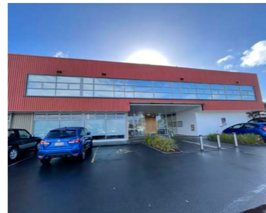
SOUTHERN FACADE - FRANKLIN FROM THE CARPARK
