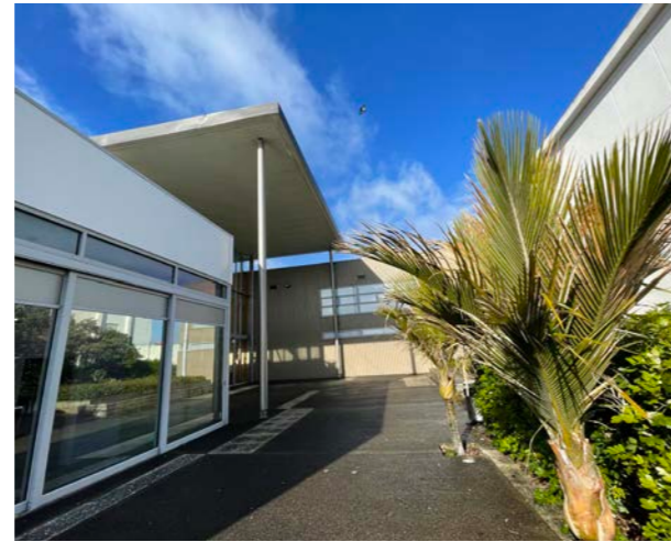
NORTHERN FACADE - FRANKLIN COVERED ROOF AREA/ LANDSCAPE
