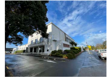
WESTERN FACADE - WAR MEMORIAL HALL
