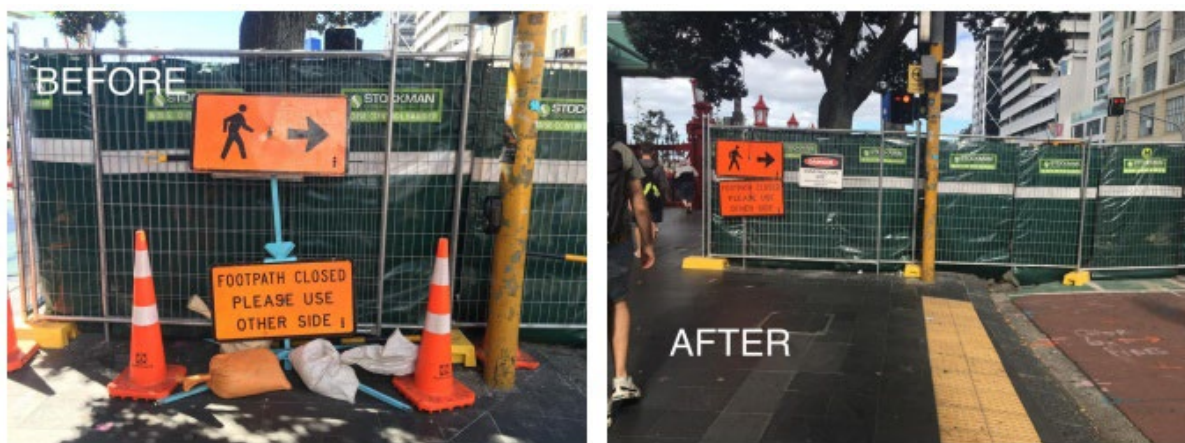
Figure 4 Example of tidy sign installation
