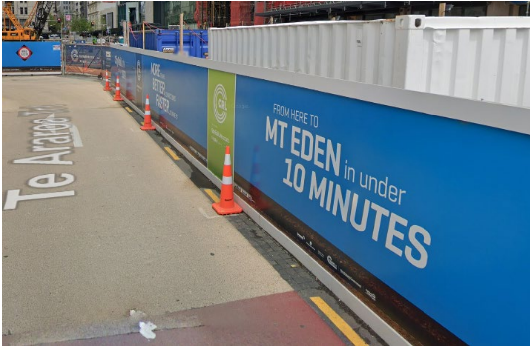
Figure 3 –Site hoarding with custom graphics for longer term establishments and major works or heavily trafficked areas. To be specified as required in tender documents.
